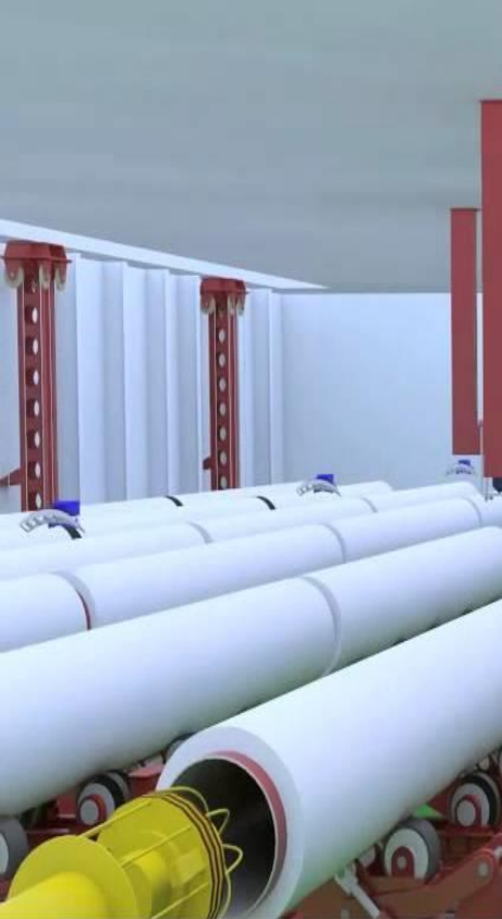
Pipe handling to firing line & Pre-heating
